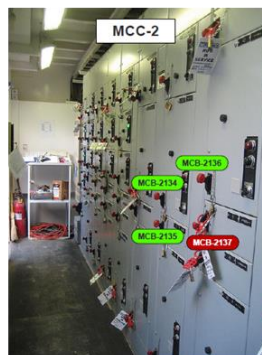
This photo is a Status Detail example showing the status of specific equipment items. Green = active; Red = LOTO
